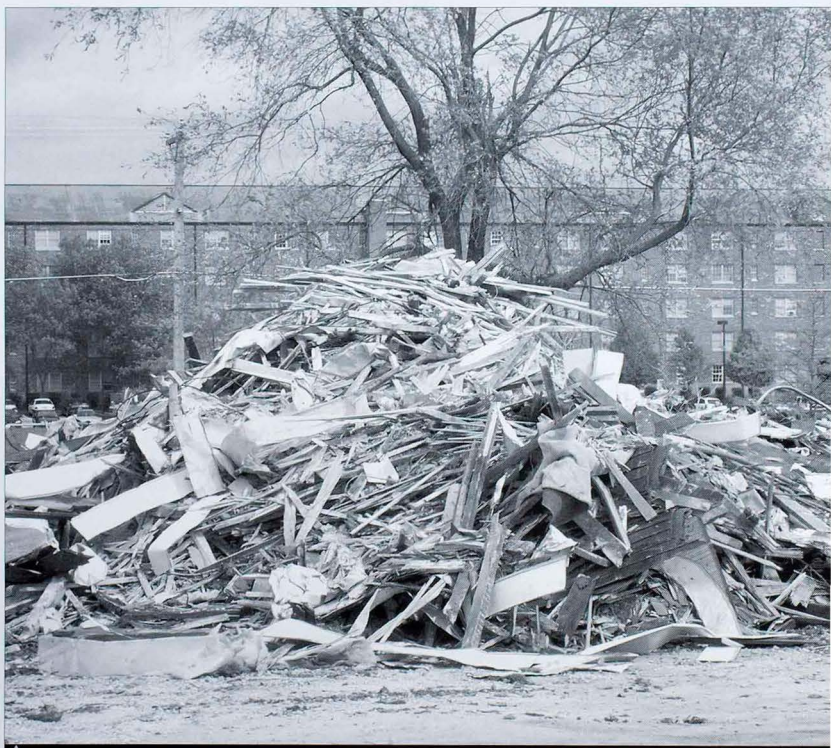
▲ The remains of the Delta Chi house lie in a pile after being demolished on April 23, 2005. Before the house was torn down it was home to four members of Delta Chi who either moved in with friends or found apartments with other Delta Chi members after the demolition.
