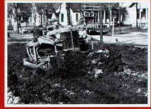
above: construction of Blanton/Nason Halls
