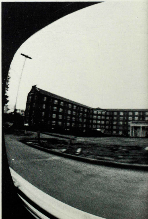
An eye's view of Centennial Hall in the early construction stages.
