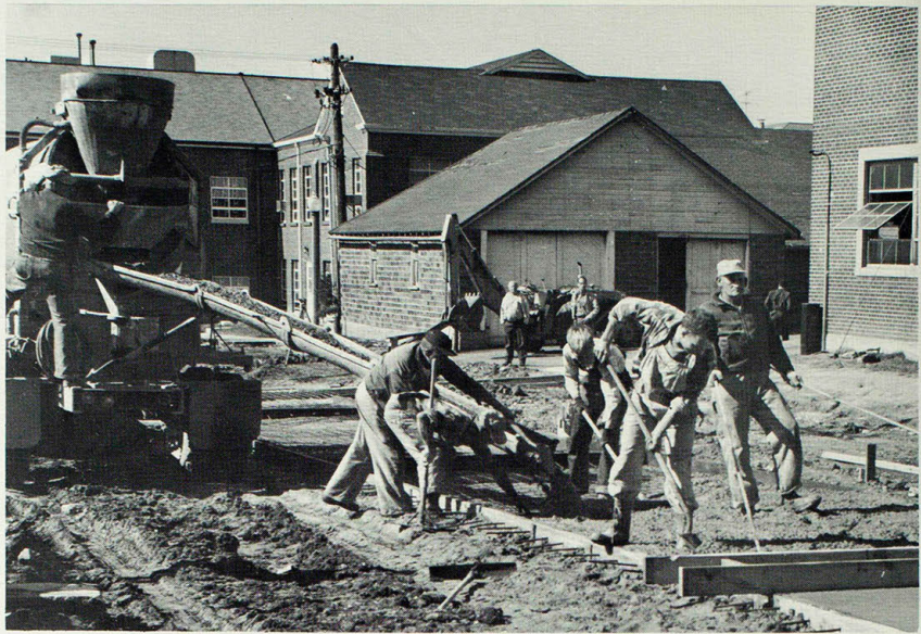
Hampered by bad weather; workmen finally start pouring much needed wide walk ways.
