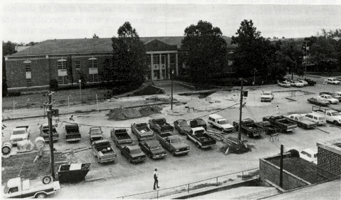
Fuel Oil Tanks Replaced —Work related to the replacement of two fuel oil tanks next to the parking lot is nearing completion. The tanks serve as a backup fuel supply to operate the power plant boiler. The work is expected to be done in mid-October at which time the Violette Hall lot will be patched and opened for parking.
