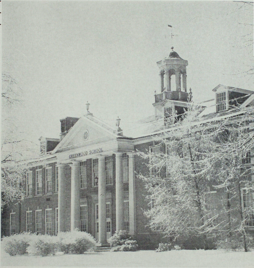
GREENWOOD DEMONSTRATION SCHOOL
