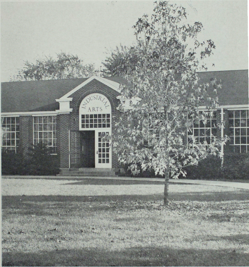
INDUSTRIAL ARTS BUILDING
