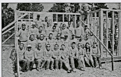
Members of Truman's Habitat for Humanity chapter pose at the construction site of a home they are helping to build.
