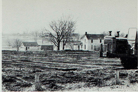
Construction finally begins on several new tennis courts south of Campbell Apartments.
