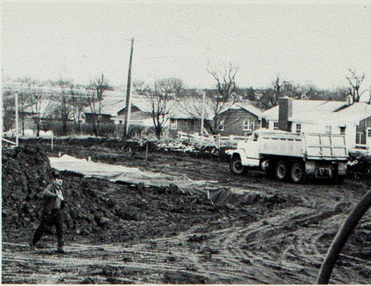
Work continues on the new Industrial Arts Building south of the Campus.
