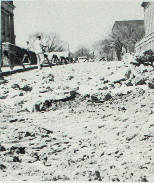
Excavation for a new heating tunnel under Marian Street connected the Pickler Memorial Library, Student Union, Science Hall, Baldwin Hall and future buildings.
